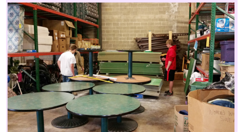
And another group from Klinsgrove United Methodist Church, Sunbury, here cutting and installing drywall.
