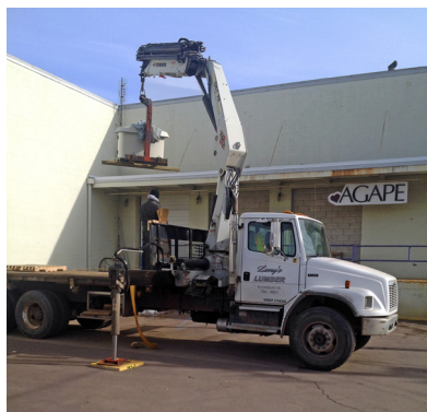
The new generator being installed.
